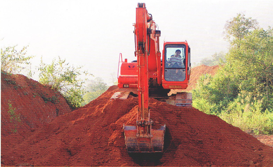
A working view of road Construction
